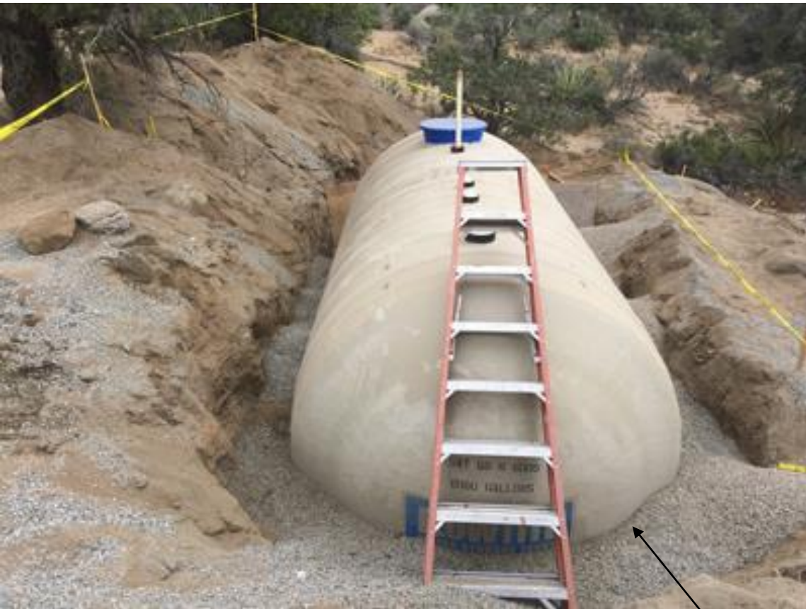
Gravel / Sand, typically 1 ft buffer around
