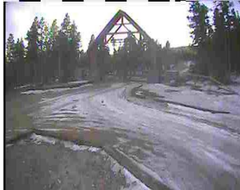
Camera 2: of Entry Approach
